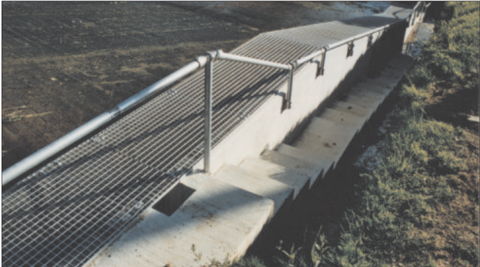
The fish pass alongside the weir at Whalesborough. Photo Chris Jewell
