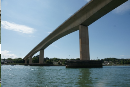
New Bideford Bridge Photos: Mike Moore
