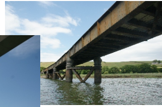
Old Railway Bridge
